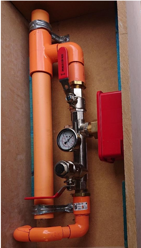
Individual sprinkler control valve
